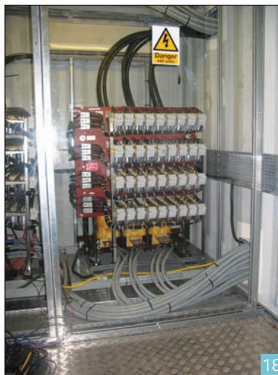
One of two 750-kW wide-spectrum harmonic filters installed on each group of combined thruster and pump load.
