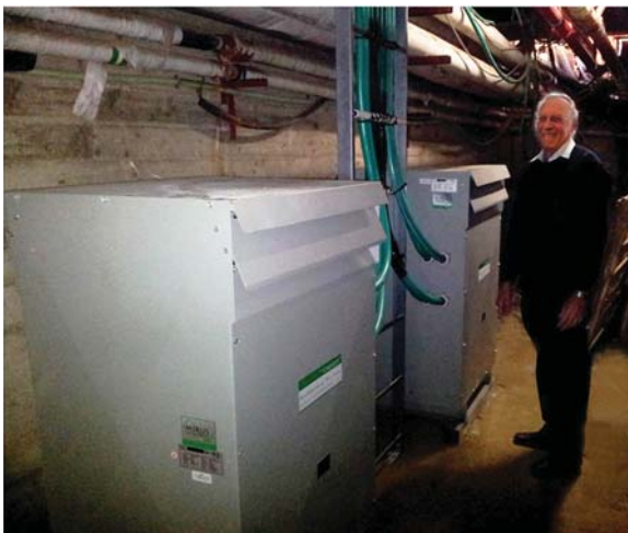
Fig. 3: Two 300HP LINEATORS at Rambam Hospital
