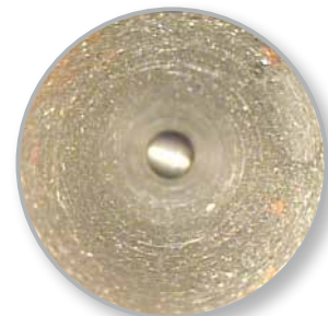
Deposits in pipe
