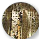
Cracks due to heat
