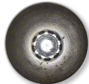
Inspection of injection nozzles
